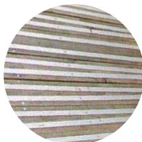
Timber Deck with Metal Inserts
