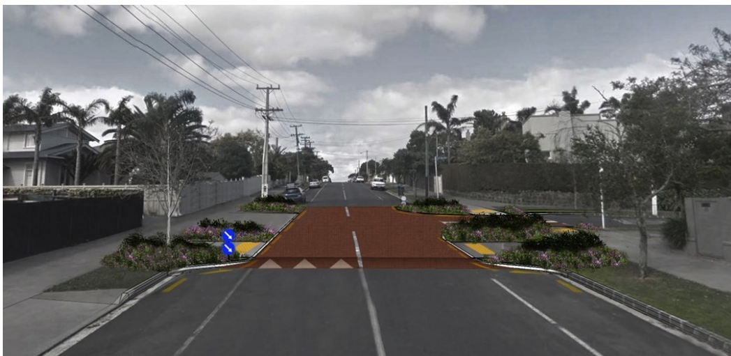
Figure 2: example of T-intersection speed table.
