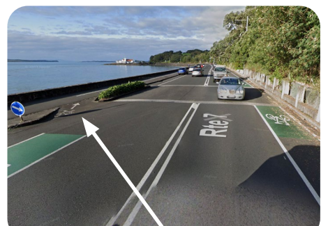
Painted cycle lane stops to gain access to the footpath.
