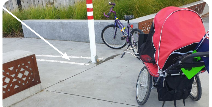
Access point - St Johns Road
