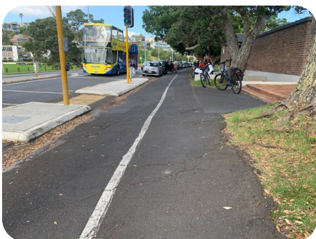
Posts encroaching on cycling section
