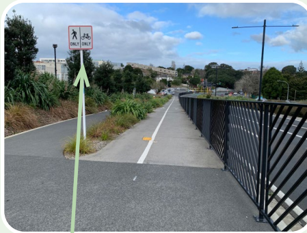
Clearly signed separation of two modes of traffic, with a general width of 2.6m overall.
