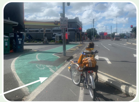
Concrete separator is angled acutely towards a cambered transition. This resulted in a cyclist tipping up.
