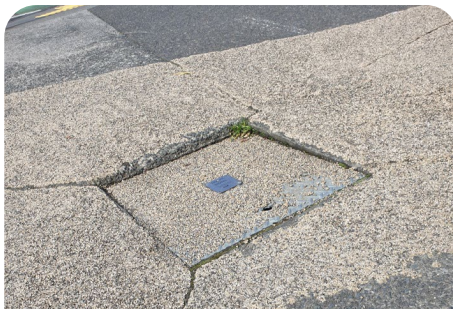
Drain is inset, making it a trap for wheels
