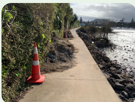
Landslip with no warning
