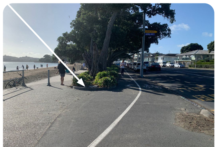
Cycleway and footpath split - no signage
