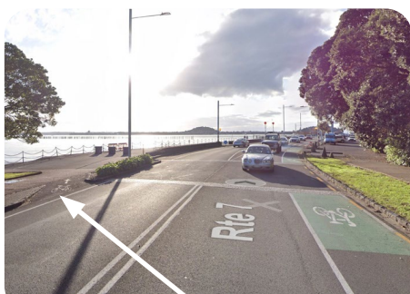
Painted cycle lane moves onto footpath suddenly
