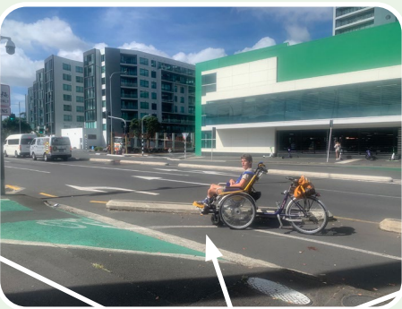
Concrete separator is angled acutely towards a cambered transition. This resulted in a cyclist tipping up.
