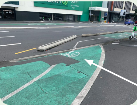
Concrete separator is angled acutely towards a cambered transition. This resulted in a cyclist tipping up.
