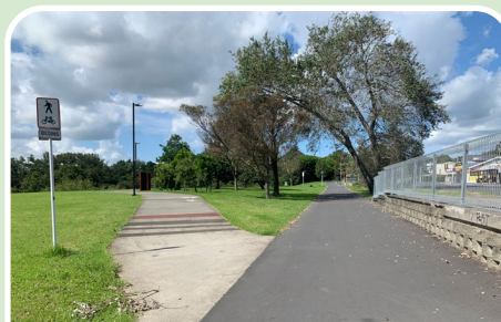
Footpath split - only Cycleway Begins sign
