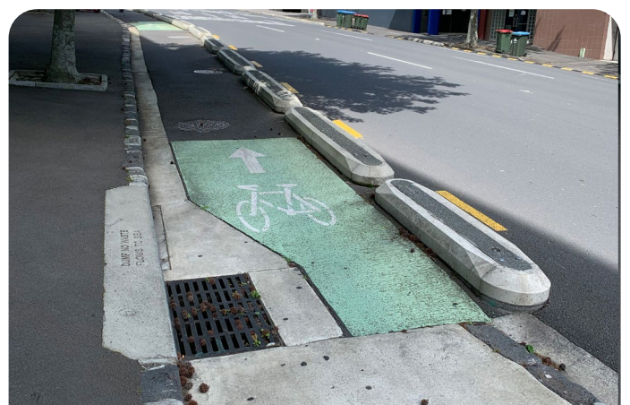
Typical drain causing hazard to trikes and sharp turn from footpath.
