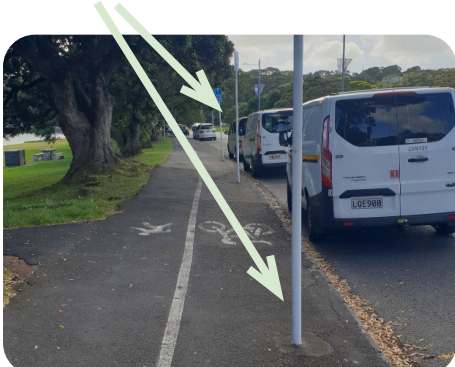
Posts encroaching on cycling section
