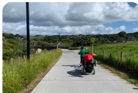
Slow down signage
