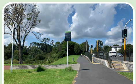
Signage indicating Waterview Shared Path on the other the path fork from opposite direction.
