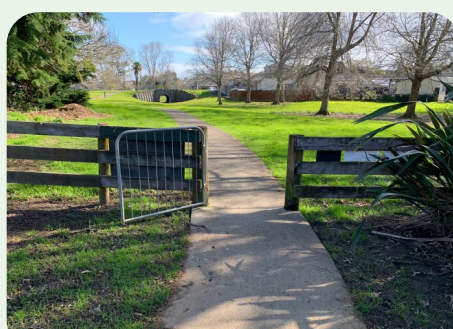
Gate post is inside the path instead of outside.
